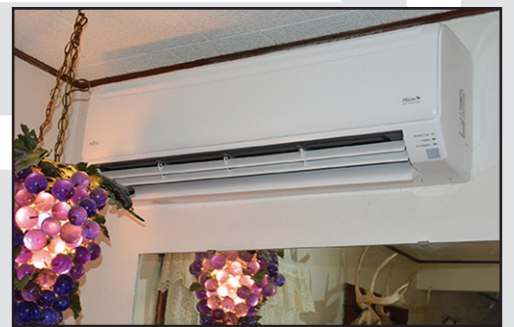
The new mini-split system.
