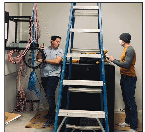
Dillon Town, left, and David Foley, work on setting up the new server vault.
