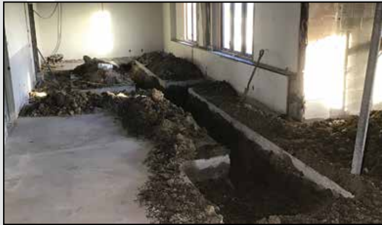
Trenches were dug in preparation for new utility lines.
