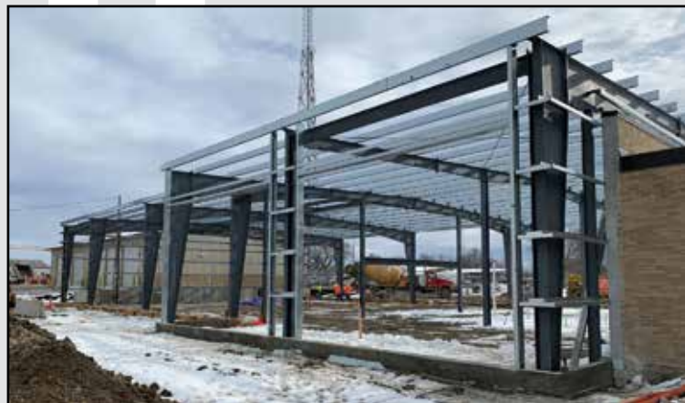
The new steel frame structure for truck and equipment storage is up. The next step is to get the structure enclosed.
